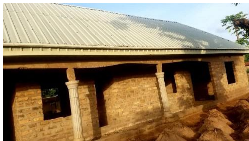
Completely roofed- but uncompleted
