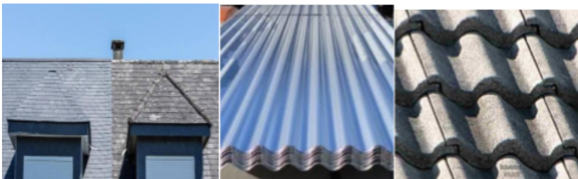
Figure 6.9: A Typical example of Slate/Asbestos, Corrugated metal and cement / concrete Roofs
