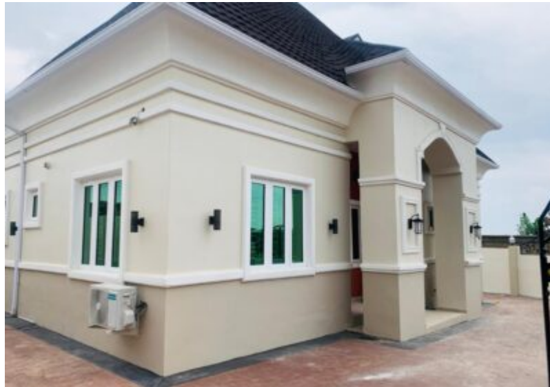
Fully completed building:
