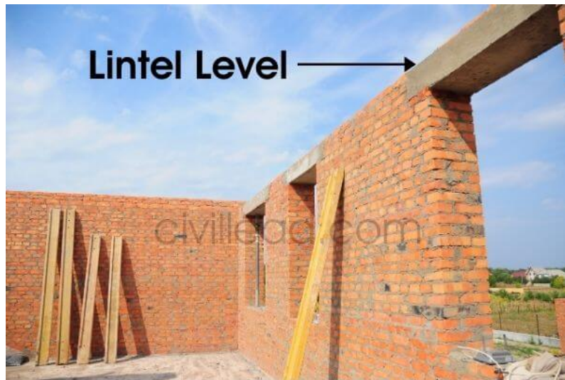
Lintel level [without roof]
