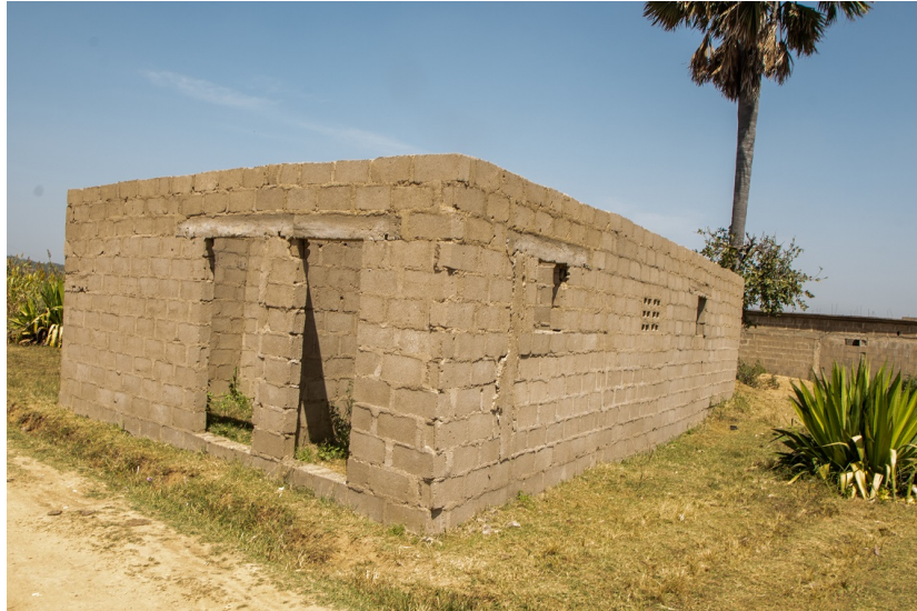
Roofing level [without roof]
