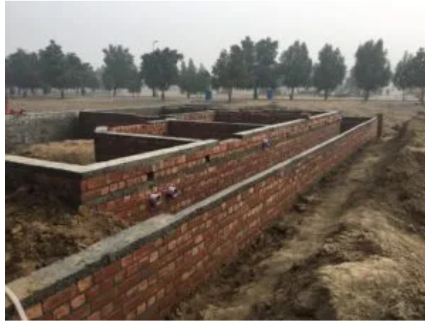
Damp-Proof Course (DPC) level
